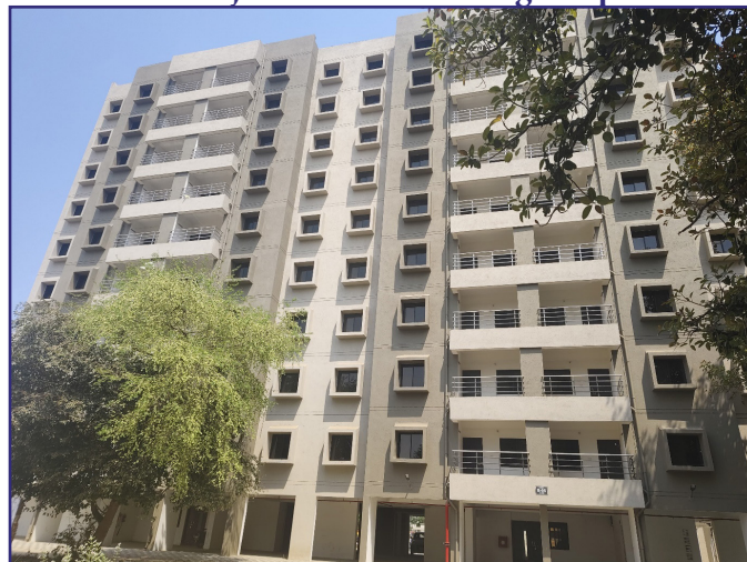
Fig. 1: Multi-Storey Residential Police Quarters Reflecting the Shift towards Vertical Housing under the Gujarat Police Housing Corporation
